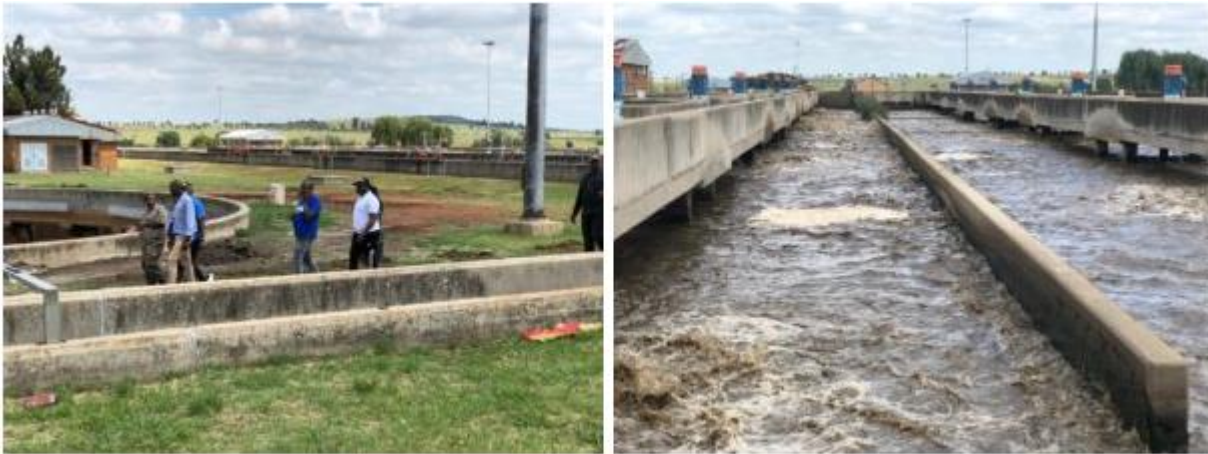
Figure 1: Sebokeng Wastewater Treatment Plant [5]
