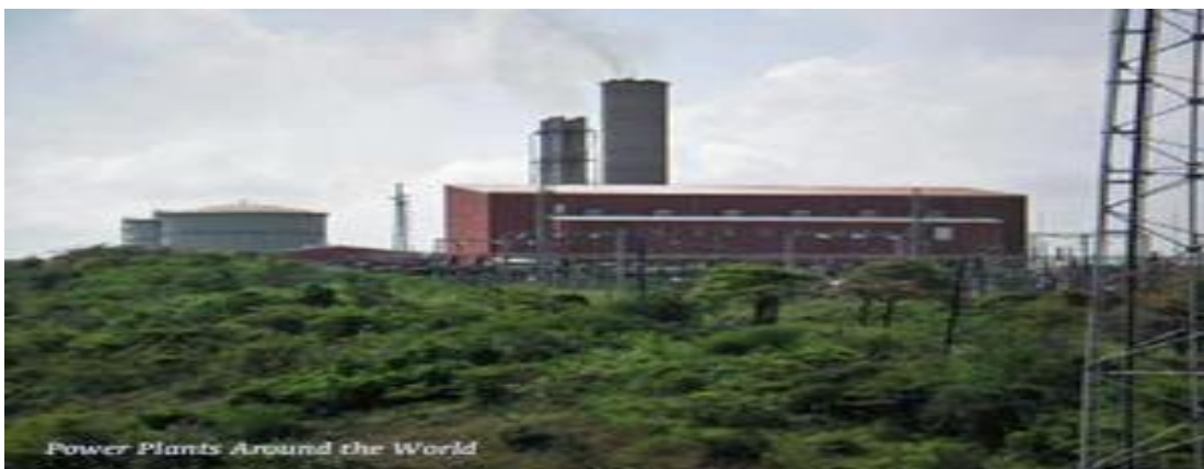
Figure 3: Kipevu 1 Power Plant [15].
